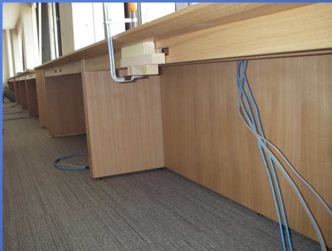
取付状況(1F)②
