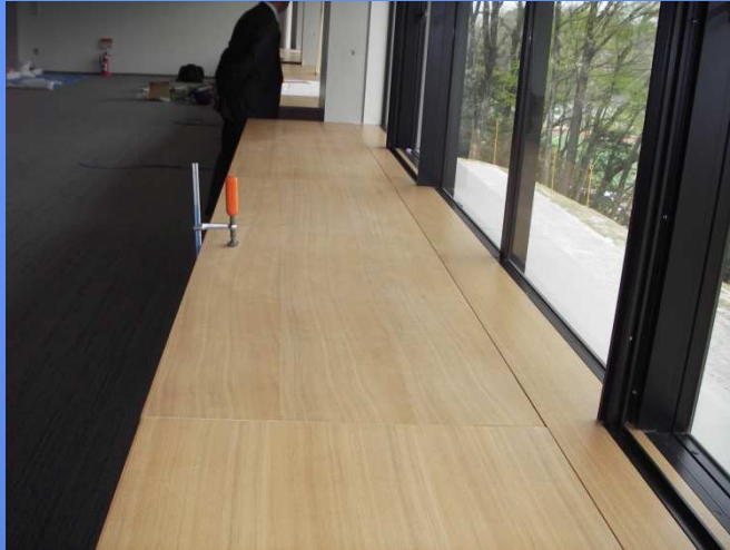
取付状況(1F)①
